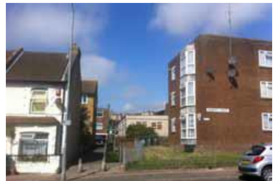
View East from Whitehawk Road (Southern Block location)
